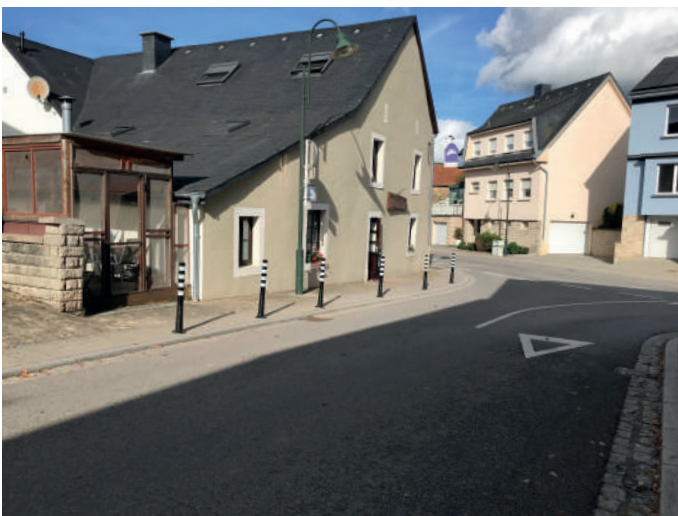
Flaxweiler, Rue Beyren - Poteaux
